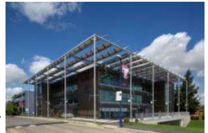
5G Innovation Centre building, University of Surrey
